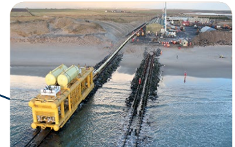
WICK BUNDLE FABRICATION, UK
