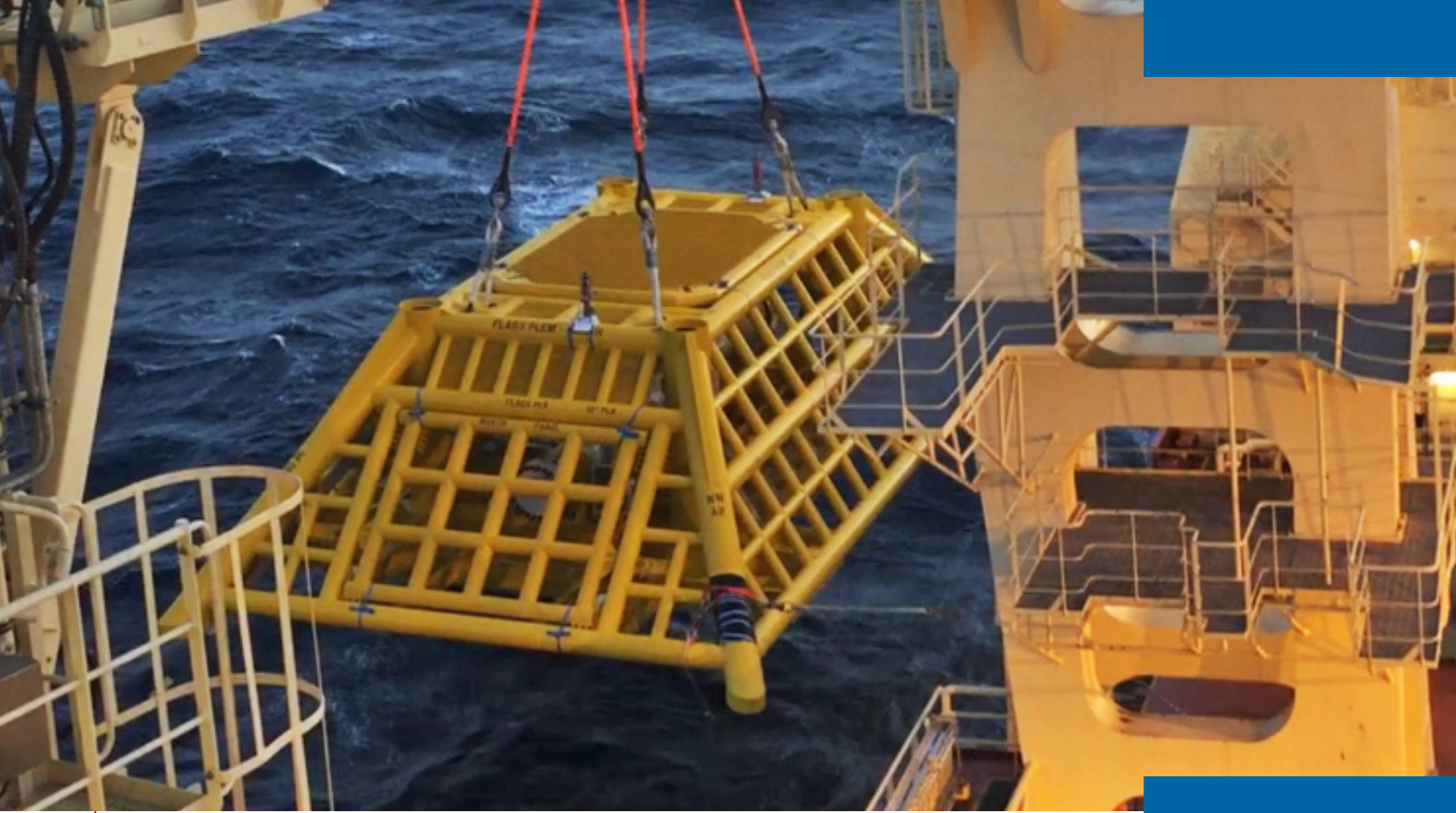
Subsea structure during installation activities
